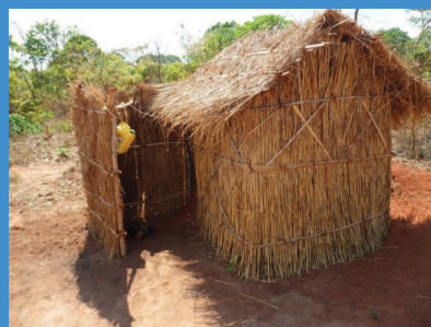
One of the 352 family latrines with hand-washing device built for displaced communities by UNICEF and IRC in Pweto.
